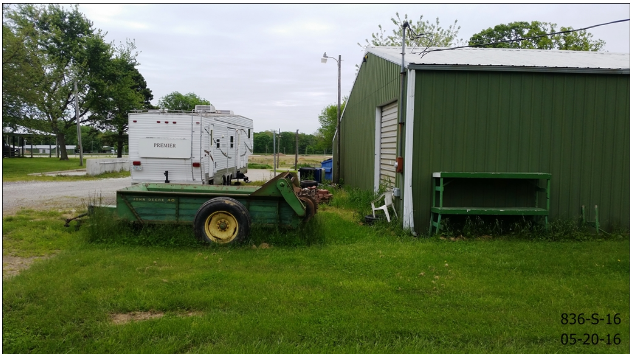
Proposed shed to be removed for parking area, from west end facing east
