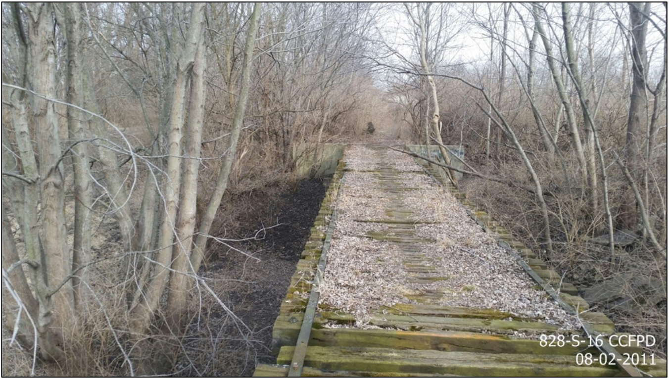
At Salt Fork River crossing, facing east
