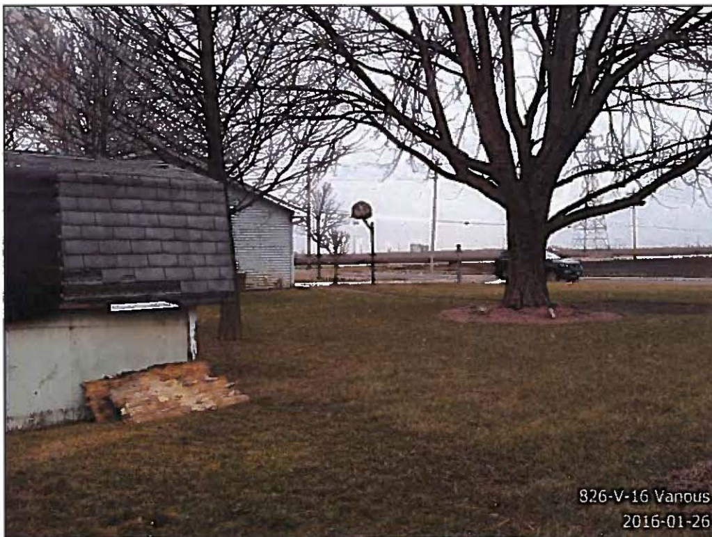
Existing shed from SW corner facing NE toward petitioners' residence
