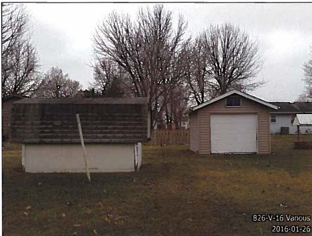
Existing shed (left) and neighbor's shed on west property line
