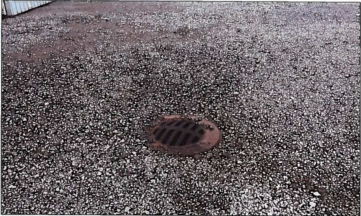
Catch basin near ditch
