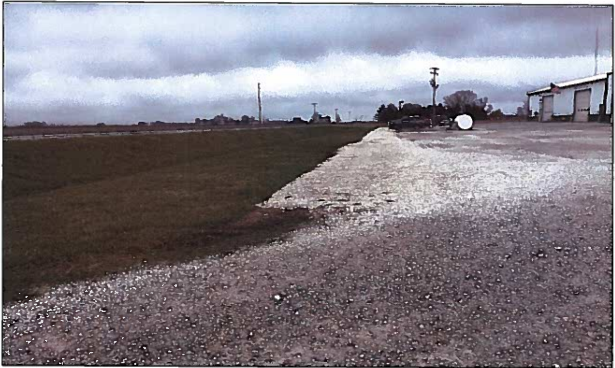
Northwest corner of property roadside ditch
