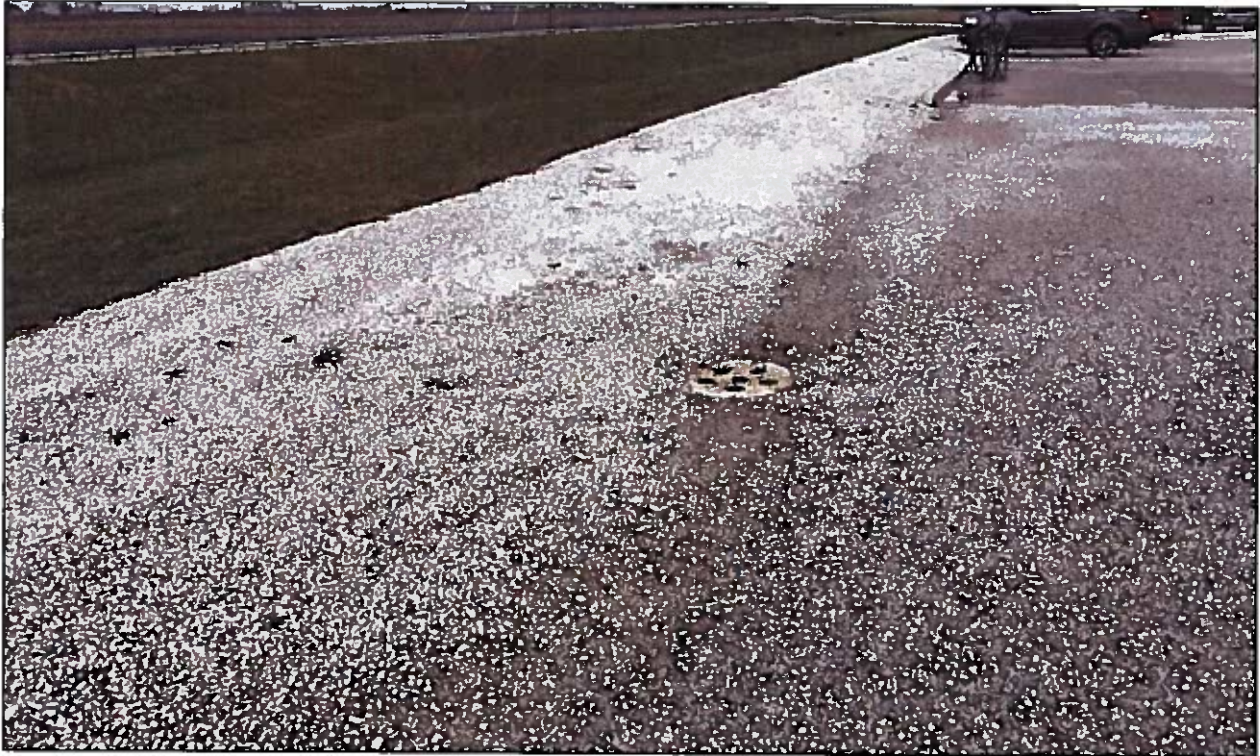
Catch basin in north parking lot
