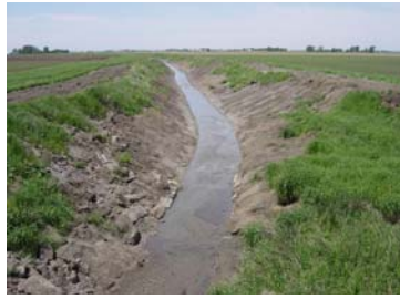
May 2005: After ditch maintenance work.
