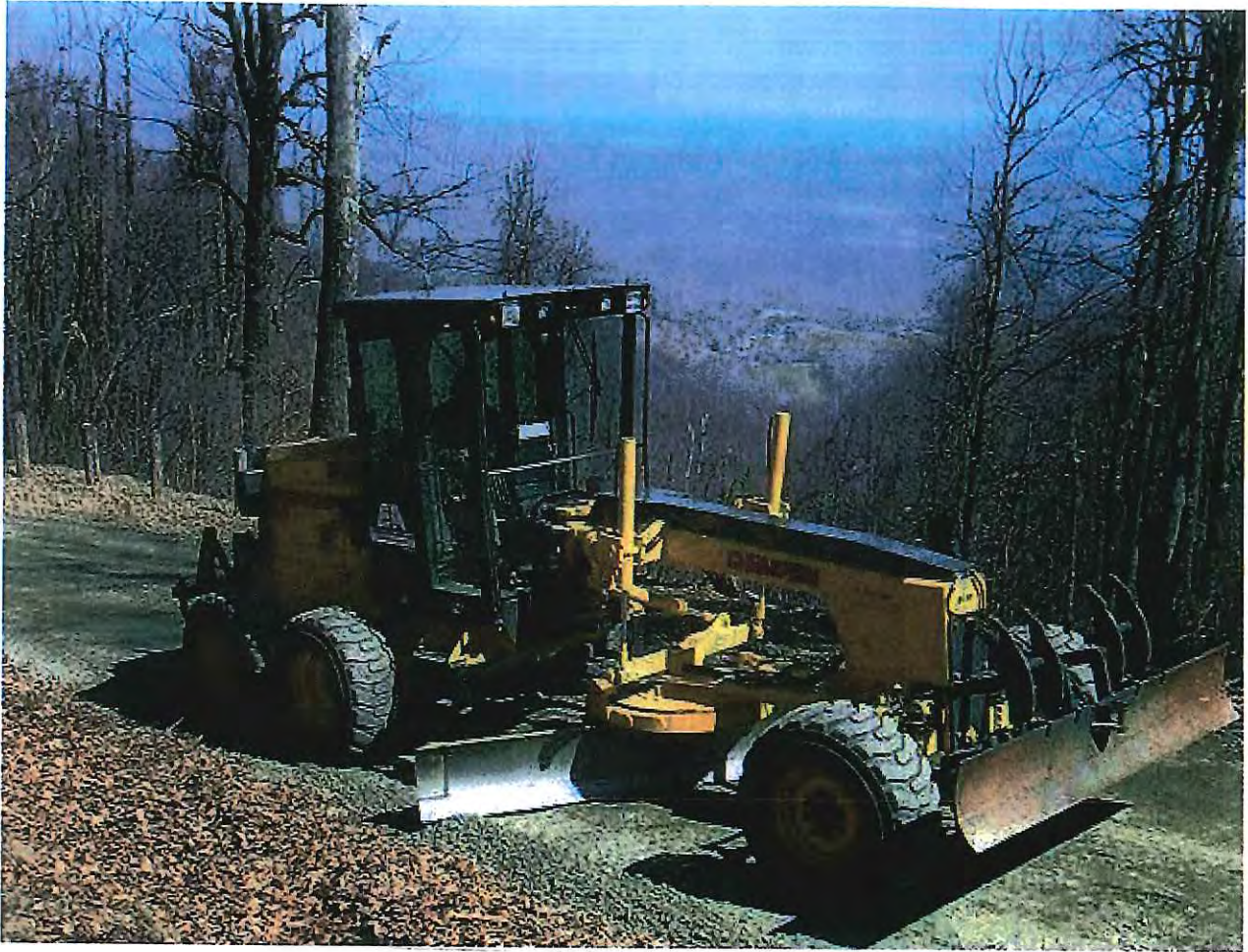
Fine Grading Equipment
