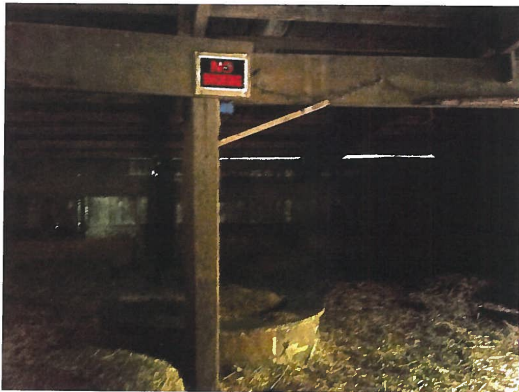
East Barn interior
