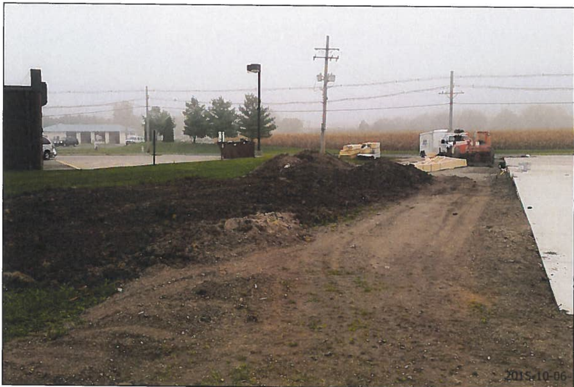
50 foot wide property west of subject property
