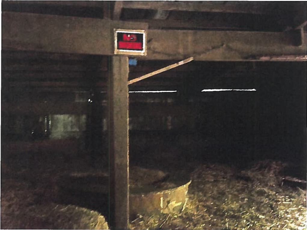
East Barn interior
