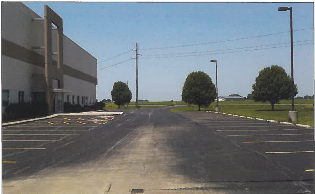
Northeast end of north parking lot facing northwest toward property access
