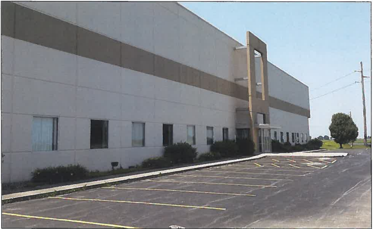
Northeast end of north parking lot facing southwest toward building entrance
