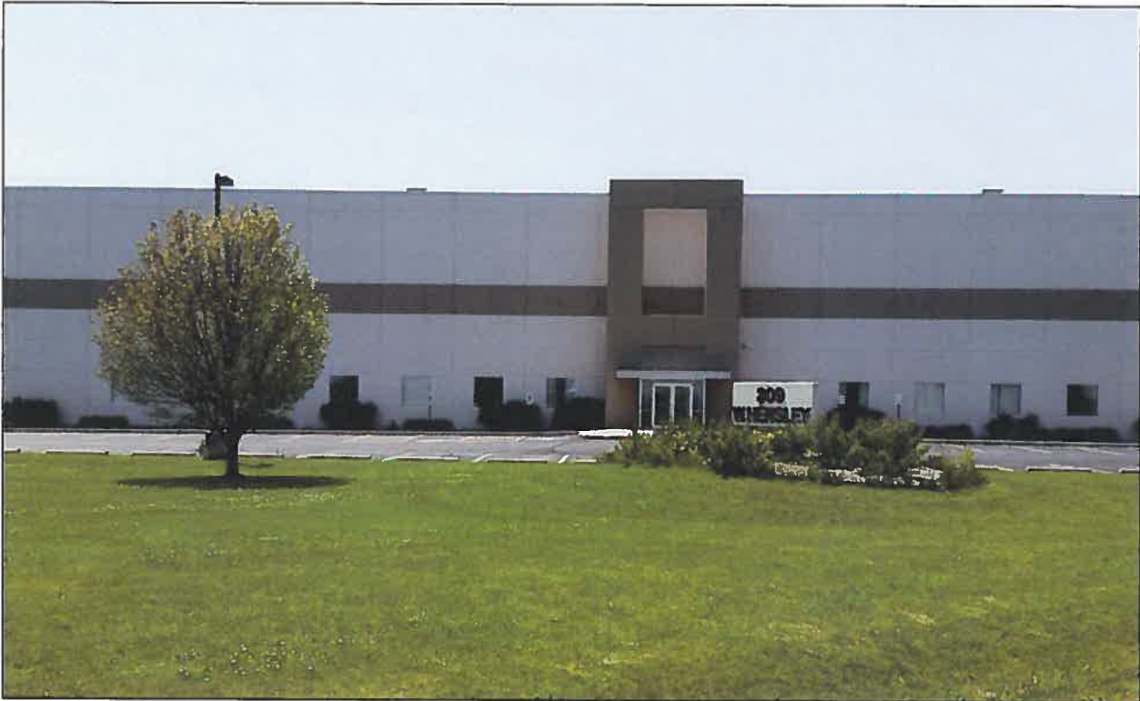
From Hensley Road, facing south
