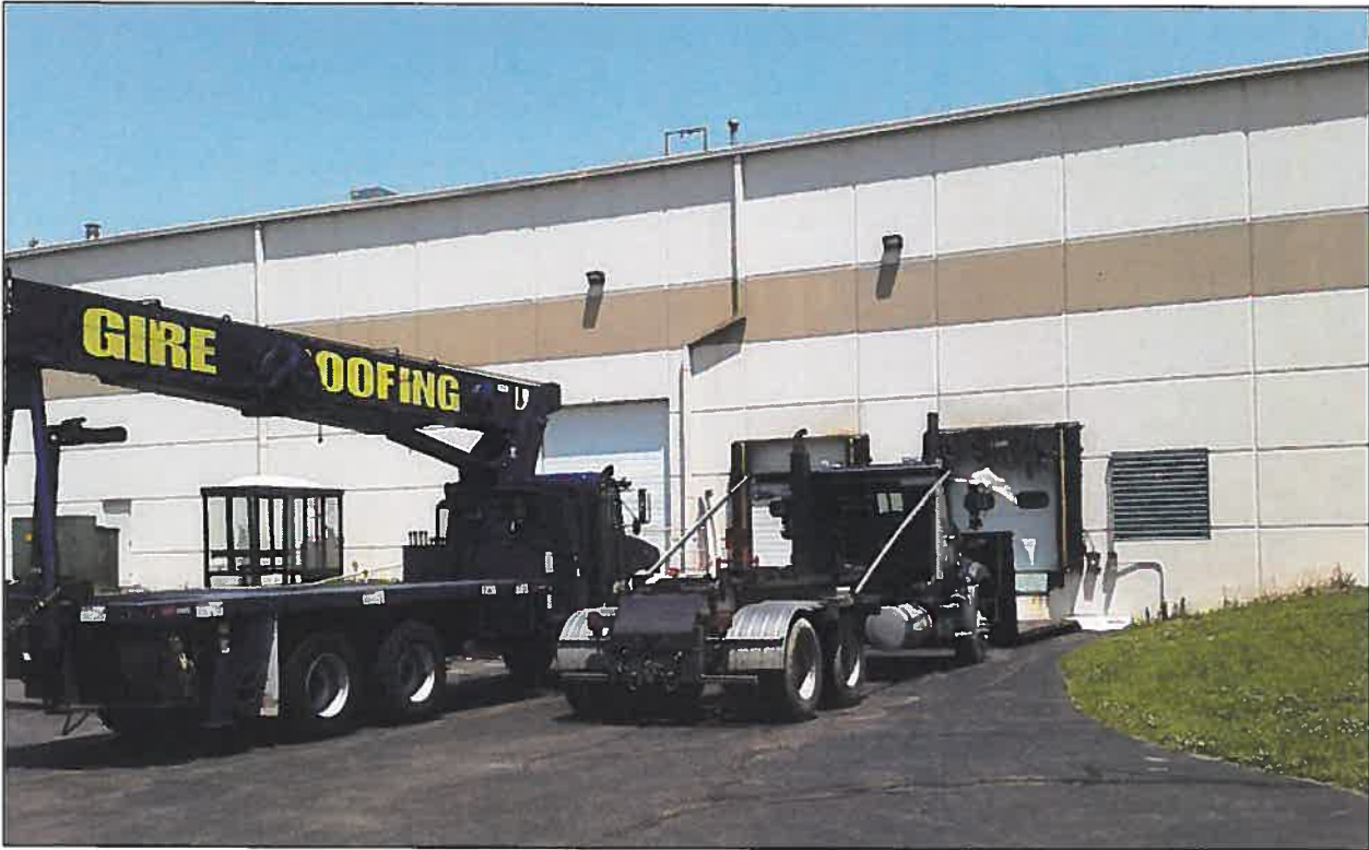
South end from parking lot, facing north
