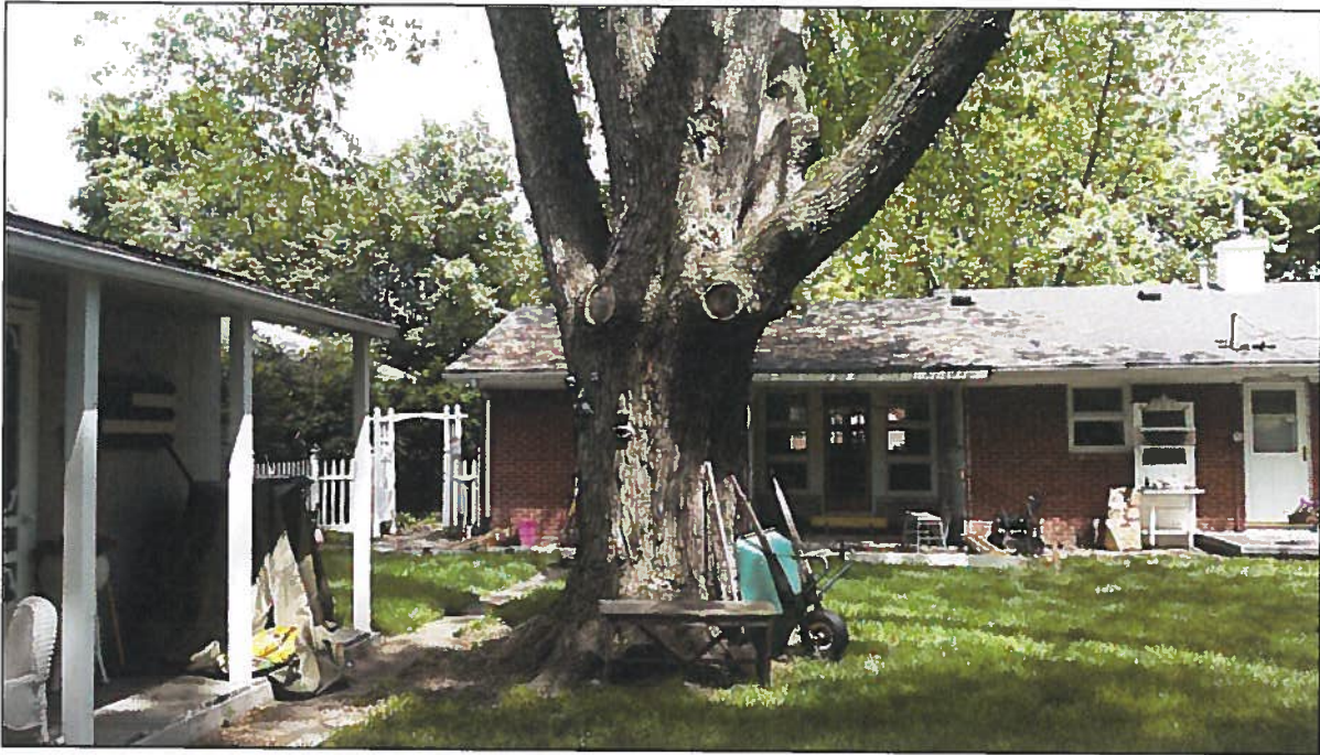
Facing north – tree in front of shed limiting its relocation
