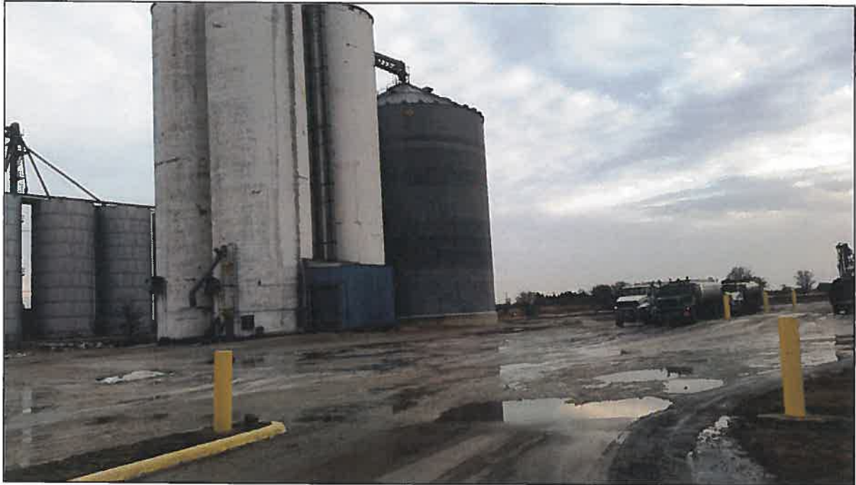
From entrance facing southeast
