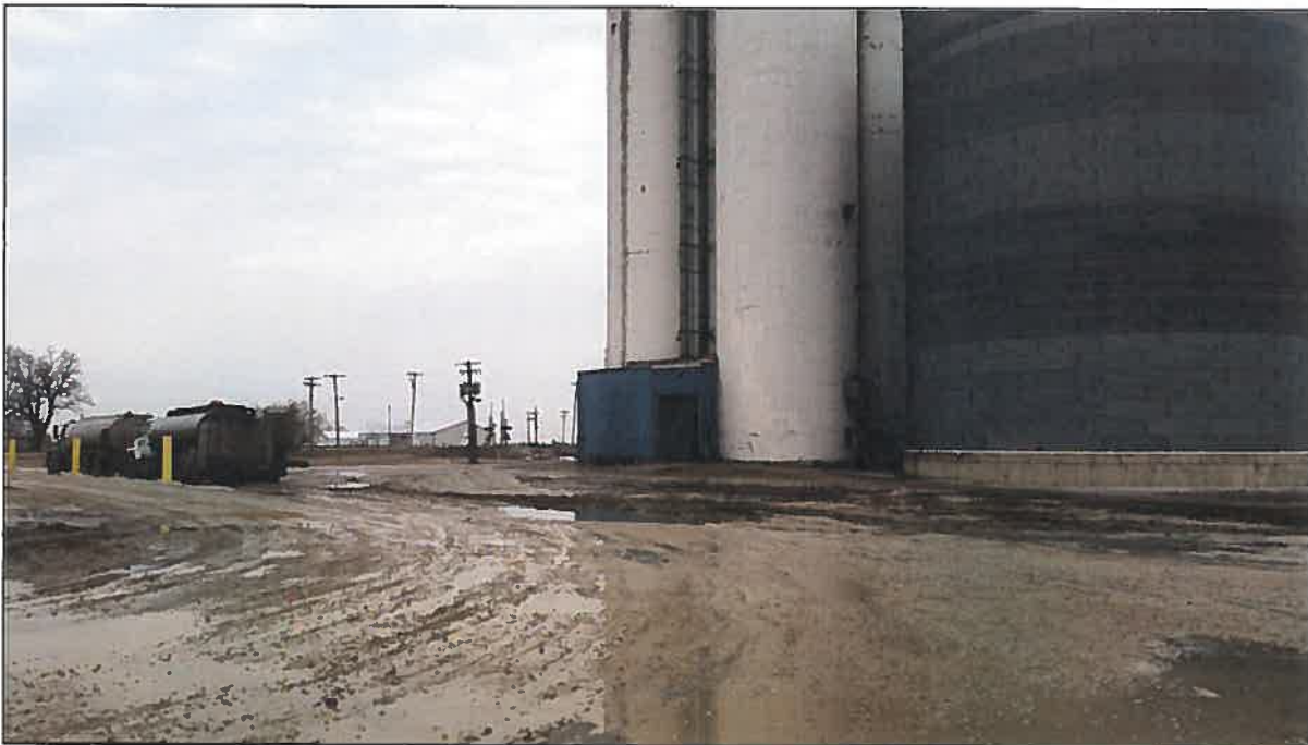
From south end of property facing northeast
