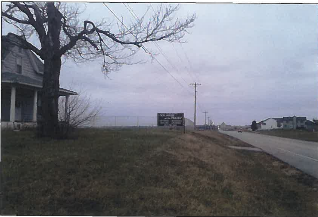
From south access driveway facing north along Staley Road – primary structure at left, fenced yard to north, business sign
