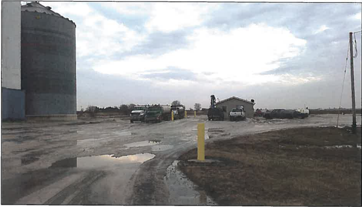
From entrance facing south
