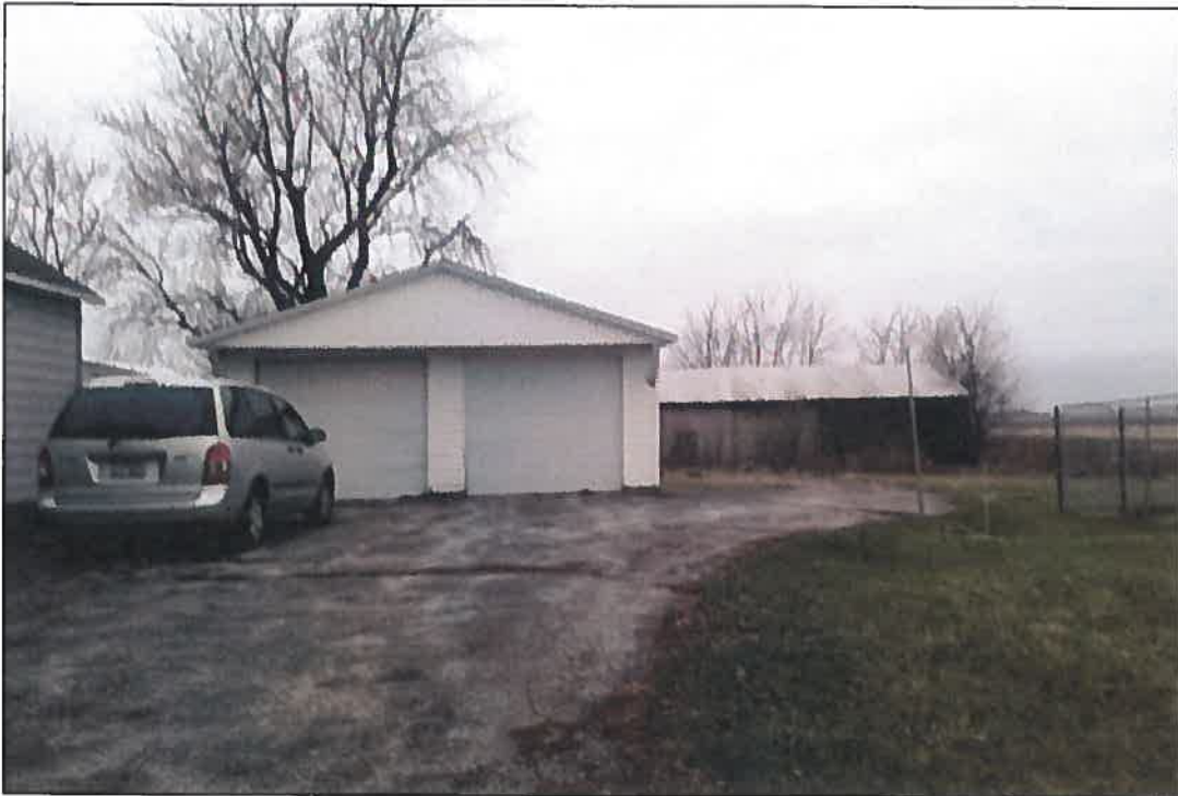
Principal structure, garage, outbuilding (to be demolished) and fenced area from north access drive facing west
