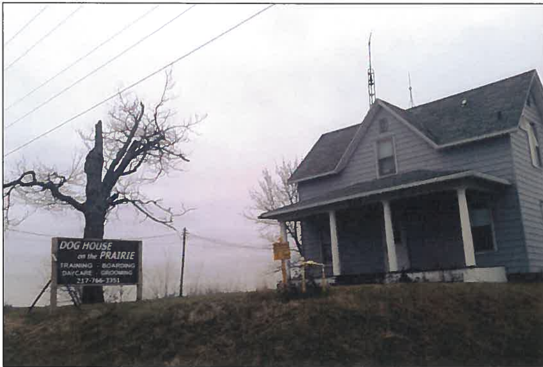
Principal structure (residence and indoor kennel) from north access drive facing SW
