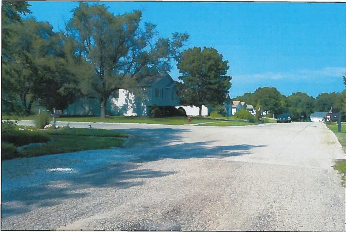
From Karadan facing NE – intersection at Summit Ridge Road (residence is on left, not shown)
