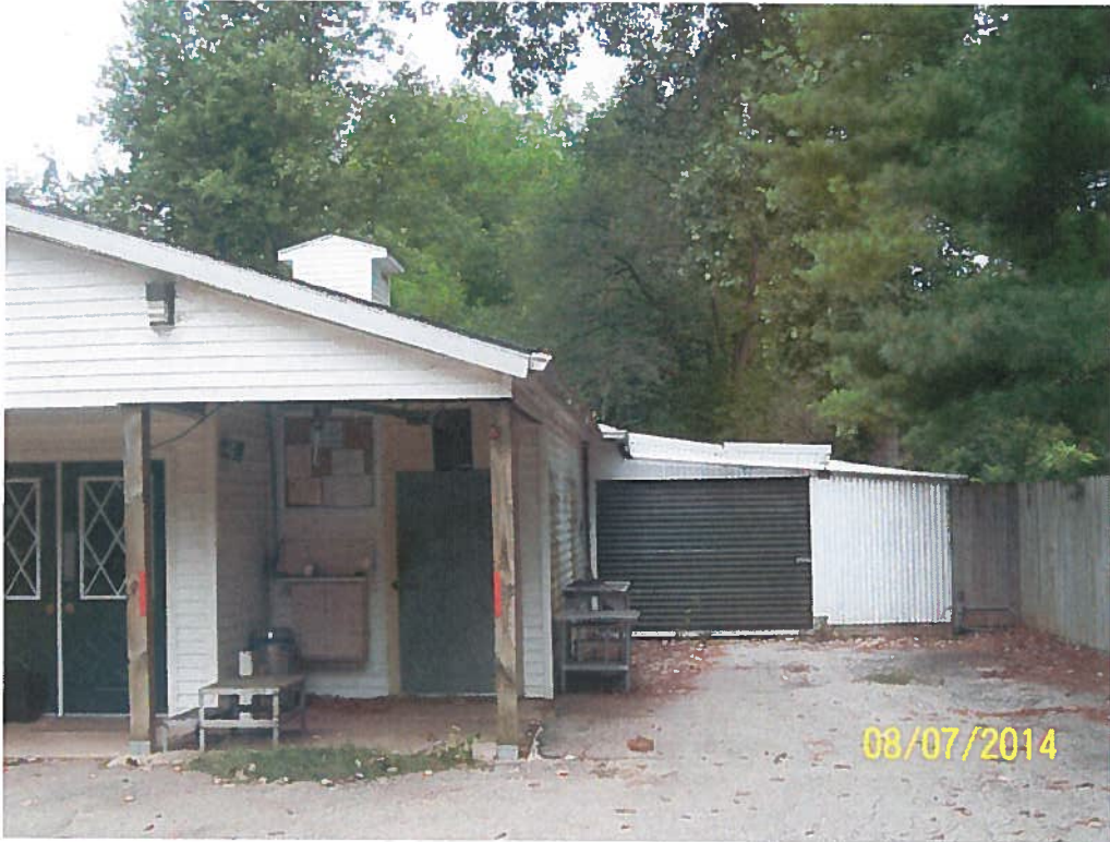
Exterior lighting on Business building
