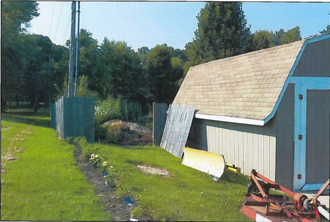
From Karadan facing NW - old shed
