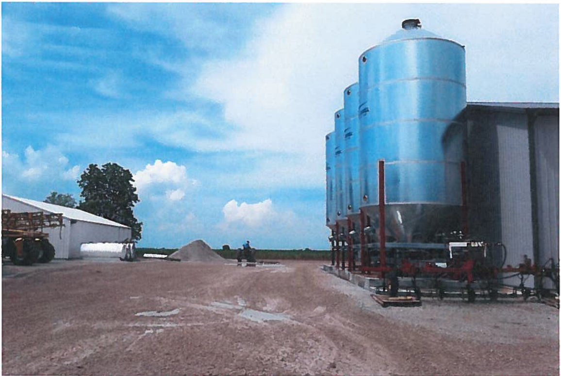
Middle of property facing N
