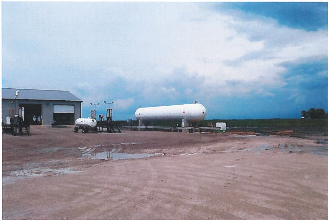
South end facing NE
