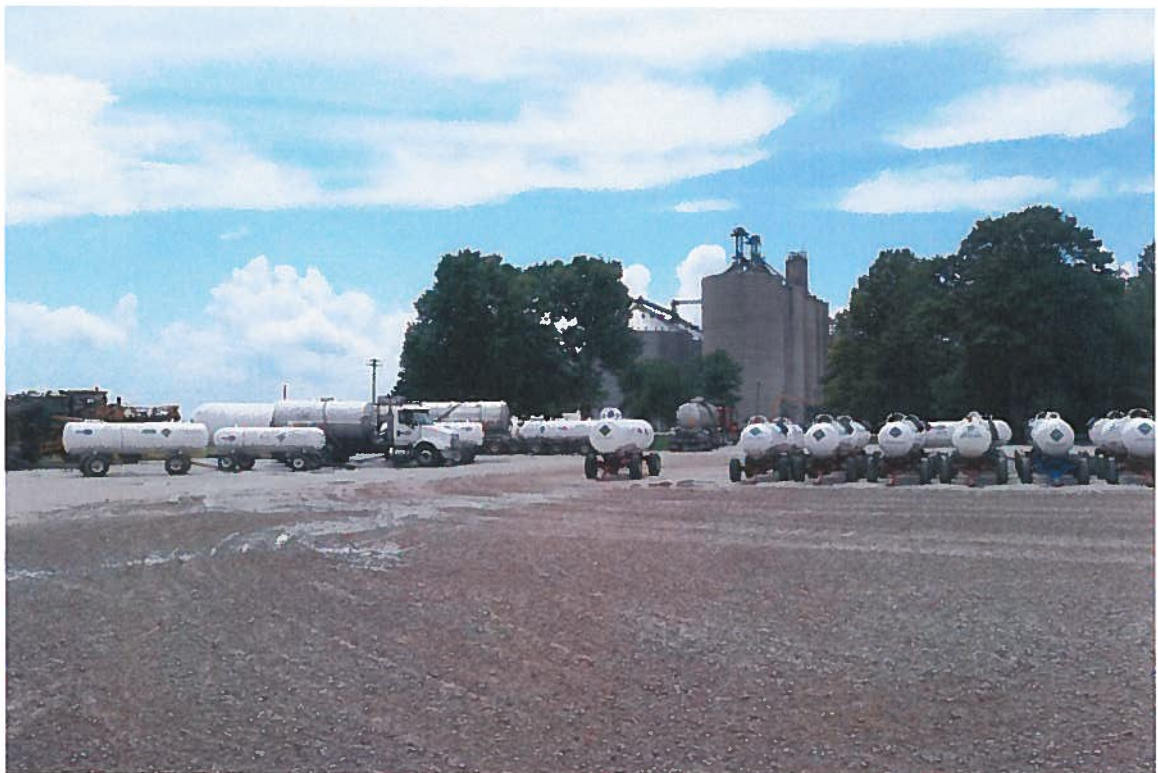
East end facing W
