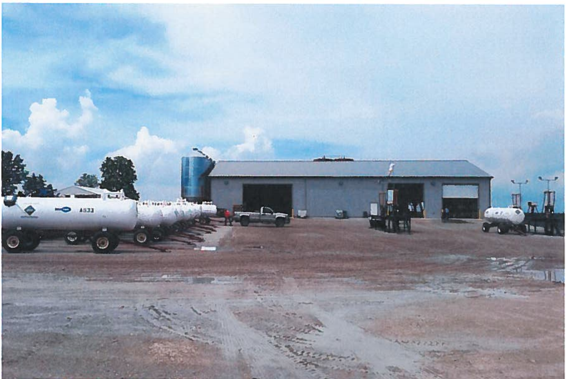
South end facing N
