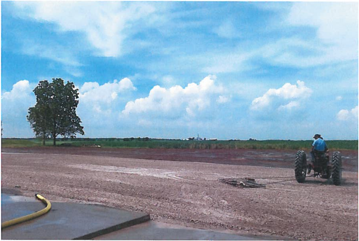
North shed facing N
