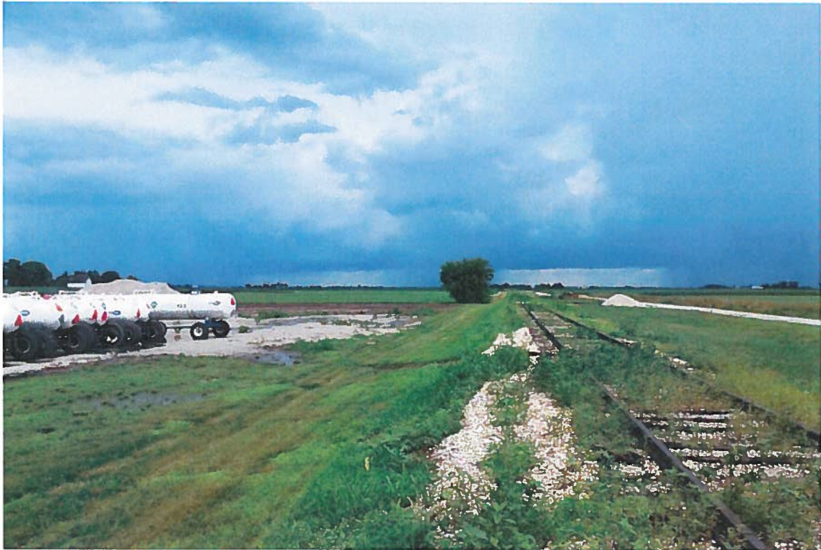
On railroad tracks facing E
