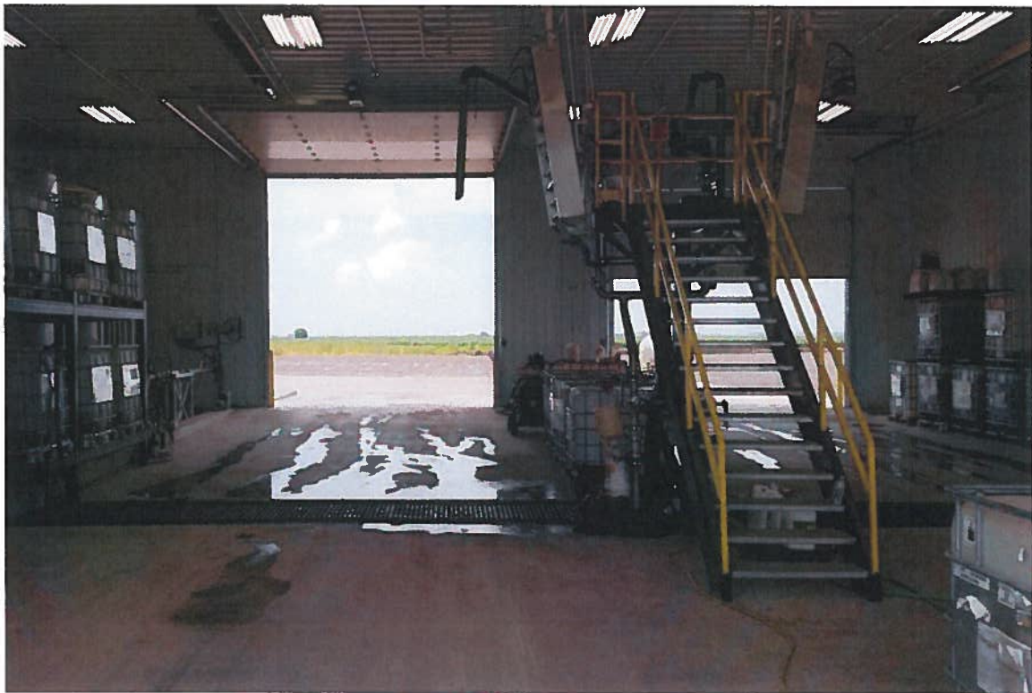
North shed facing N
