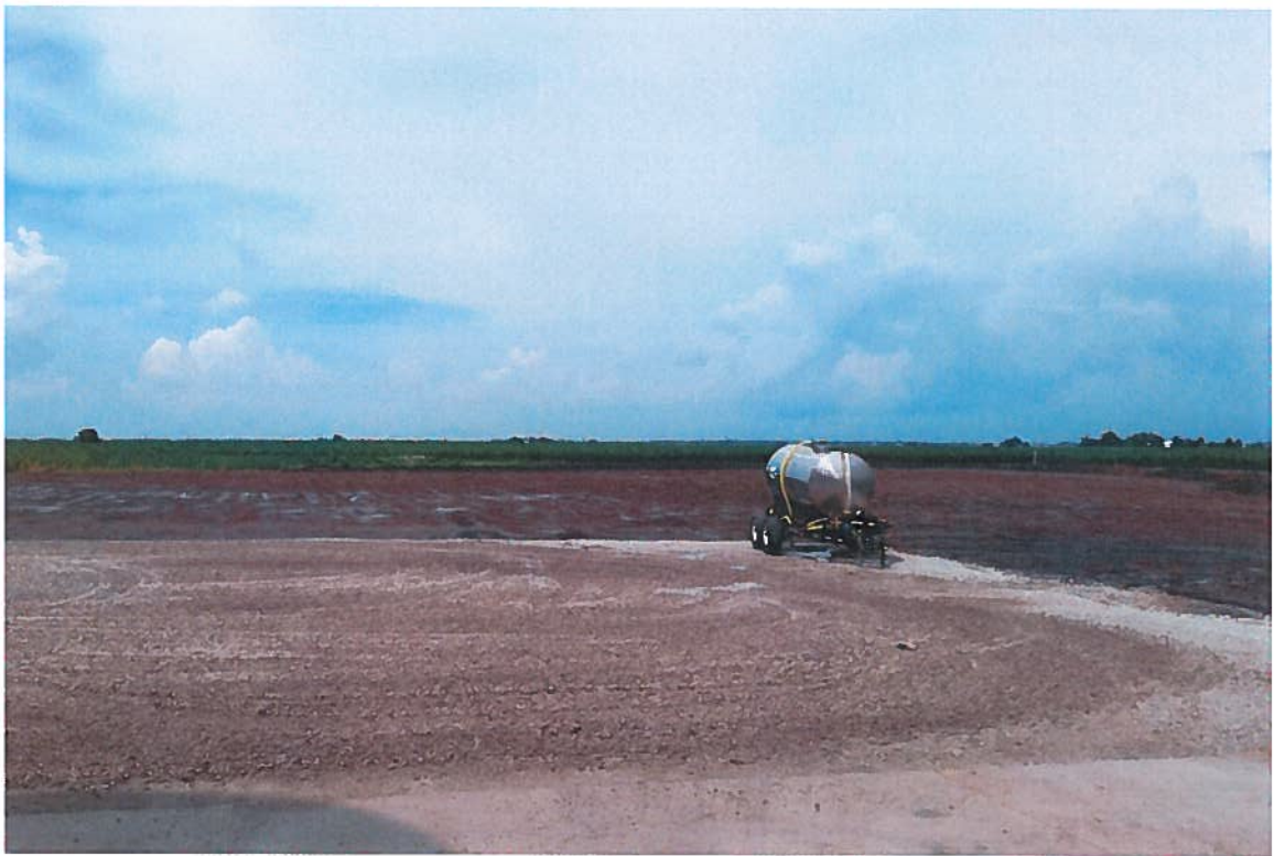
North shed facing N
