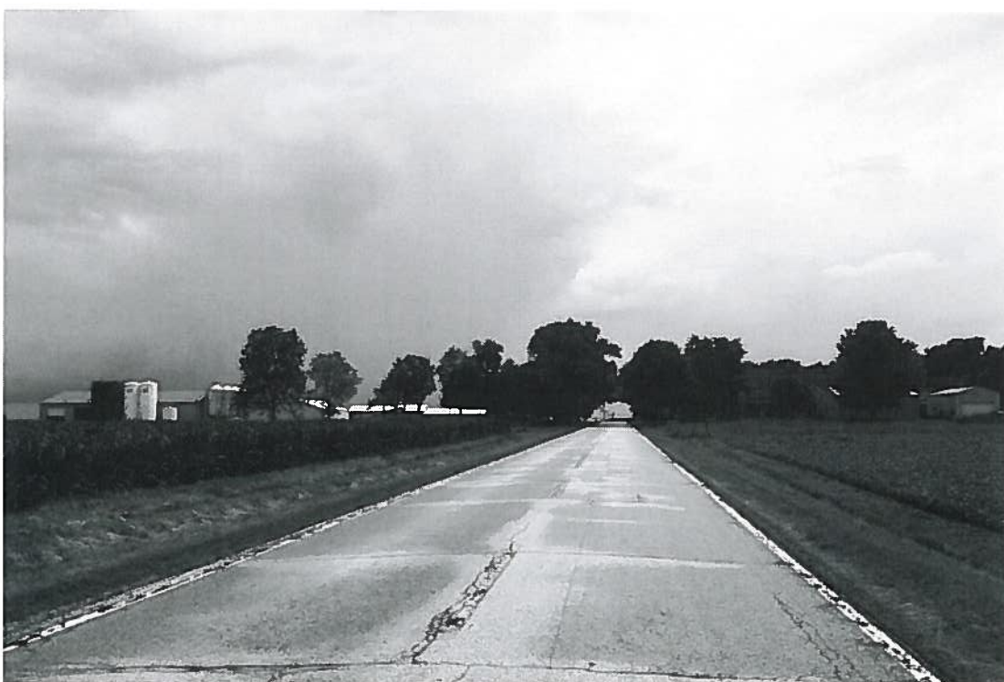
Road facing S, United Prairie on left
