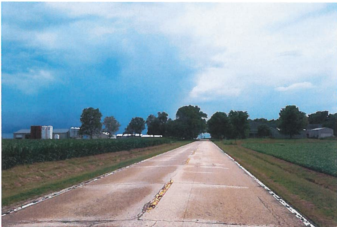
Road facing S, United Prairie on left
