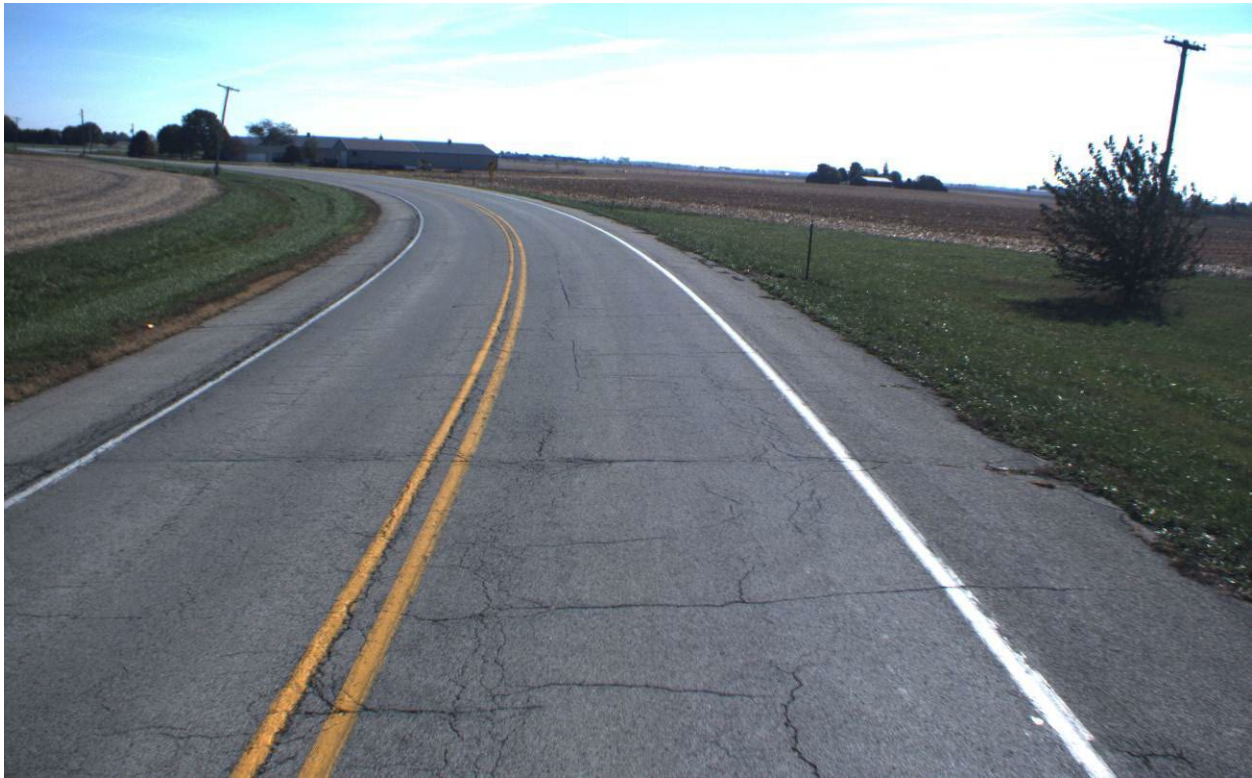
Figure 2. Digital images taken every 15 feet show pavement distresses and roadside assets.
