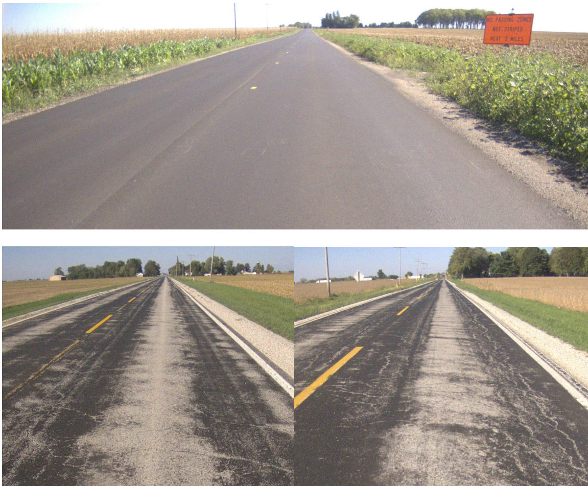
Figure 1. Champaign County's PMS optimizes the expenditure of construction funds over the long-term by choosing the appropriate treatment and timing for road improvements, such as the CH 15 rehabilitation from SR 130 to Sidney in 2021 (top) and the Cold In-place Recycling (CIR) that will take place in 2023 on CH 12 (bottom left) and CH 24 (bottom right).
