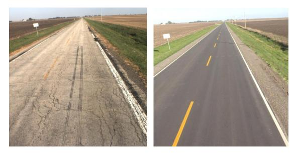
Figure 1. Champaign County's PMS optimizes the expenditure of construction funds over the long-term by choosing the most appropriate treatment and timing for road improvements (County Highway 23, pre- and post-2017 construction).
