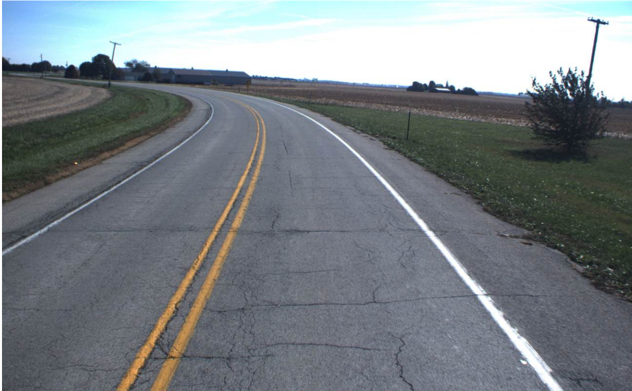
Figure 2. Digital images show taken every 20 feet show pavement distresses and roadside assets.
