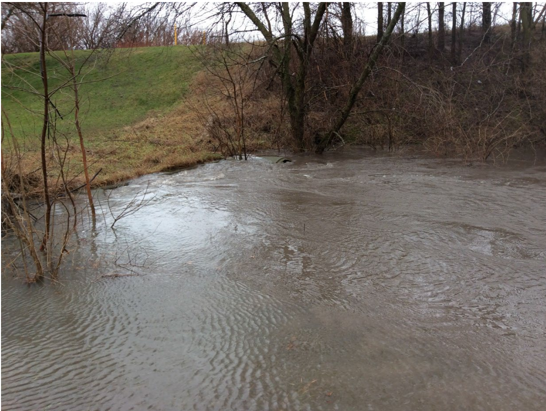
This is the same culvert taken the same day as the first photo of Corky's Auto. I have seen the water higher than this then the water will flow beside the culvert all the way to the other end of the culvert 700 feet away and the flooding at Corky's and Fountain Valley is very bad.
