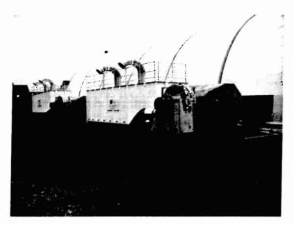
The "tent" ventilating system maintains the inside air at a lower pressure than the outside air to minimize uncontrolled releases. Air is vented to the outside through filters (shown here at Ameren's Jacksonville MGP site) that capture dust and vapors from the tar and the vehicle exhaust. The enclosure and its filtering system will significantly reduce the vapors and possibility of tar-like odors in the area. Photo taken at the Ameren Illinois Utilities MGP remediation in Jacksonville.
