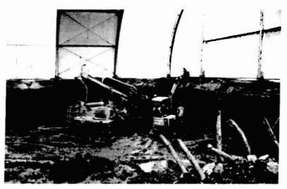
Inside the tent, specially trained workers remove source material and contaminated soil. The material is hauled away in covered trucks. Clean fill is then placed in the excavated area. Photo taken at the Ameren Illinois Utilities MGP remediation in Jacksonville.
