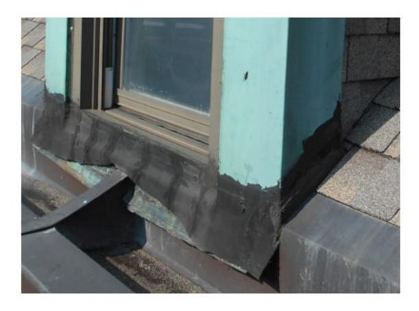
Flashing repairs needed around courthouse windows.
