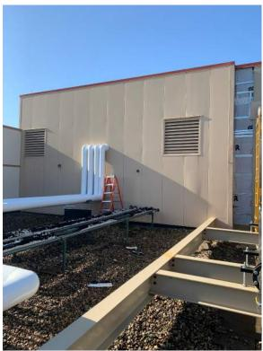
Outdoor pipe insulation has been installed.
