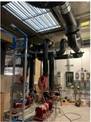
Insulated water pipe connected to pumps.
