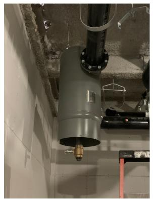
Air separators have been installed.
