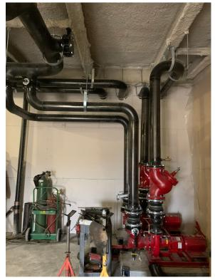
Pipes being installed to pumps.
