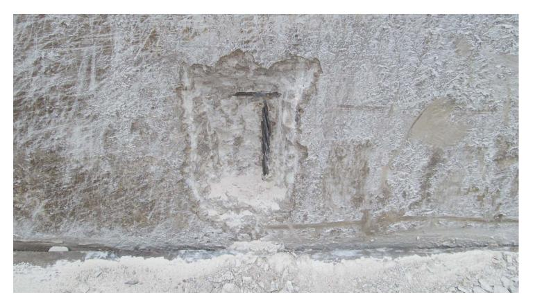
Photograph #12: The left-center prestressing strand was corrosion free.
