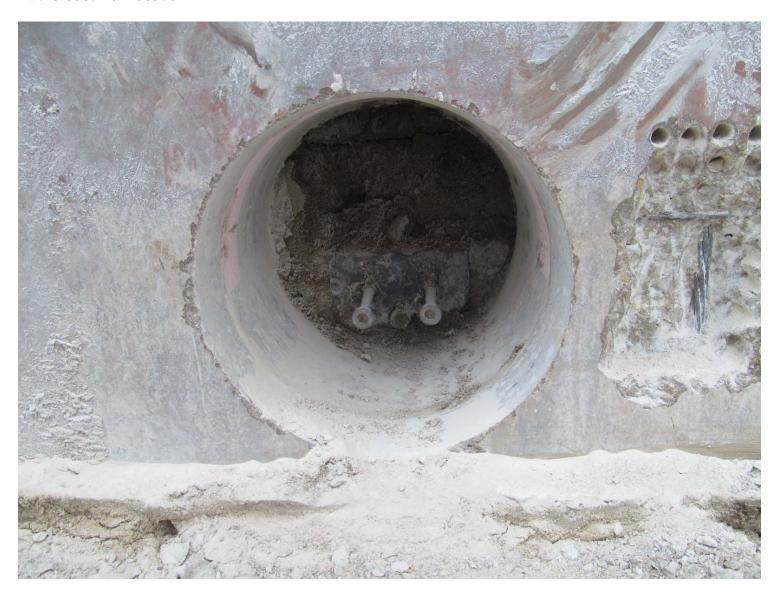
Photograph #5: The Wall Panel Base connection exhibited surface corrosion.
