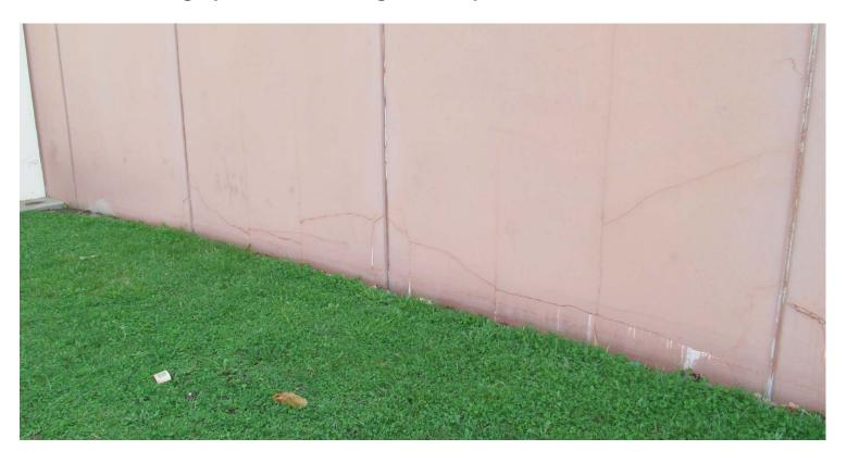
Photograph #23: Cracking at the ground line of a West Wall Panel
