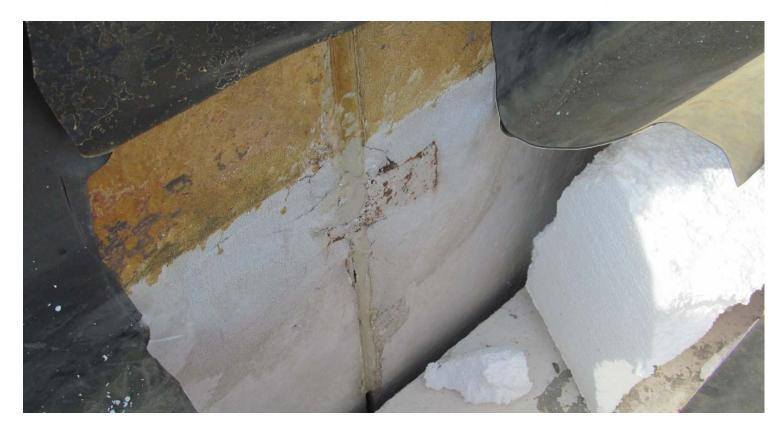
**Photograph #25: Interior Wall Panel Joint Sealant**
