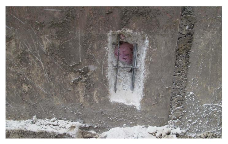
Photograph #8: The strand on the right side of the panel was corrosion free.
