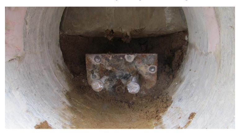
Photograph #16: The Wall Panel Base connection exhibited surface corrosion on the buried face. The steel connection is buried in moist sand below the floor.
