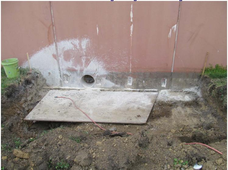
Photograph #4: Close-up of Photograph #1 showing Vertical Cracking
