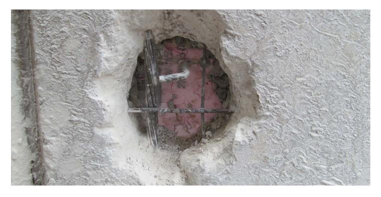
Photograph #17: The strand on the left side of the panel was corrosion free. The L-shaped tie wire is the mechanical connection between concrete layers.
