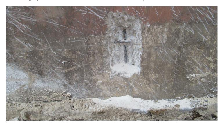
Photograph #7: The right-center strand exhibited surface corrosion.
