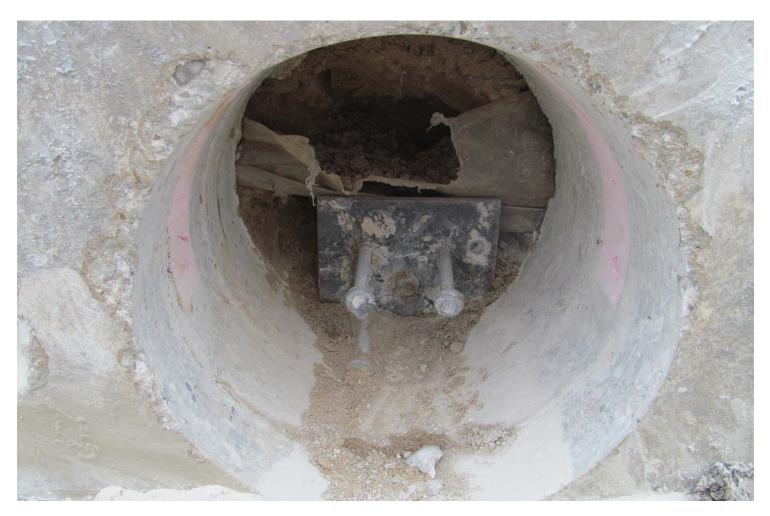
Photograph #10: The Wall Panel Base connection exhibited surface corrosion on the buried face. The steel connection is buried in moist sand below the floor.
