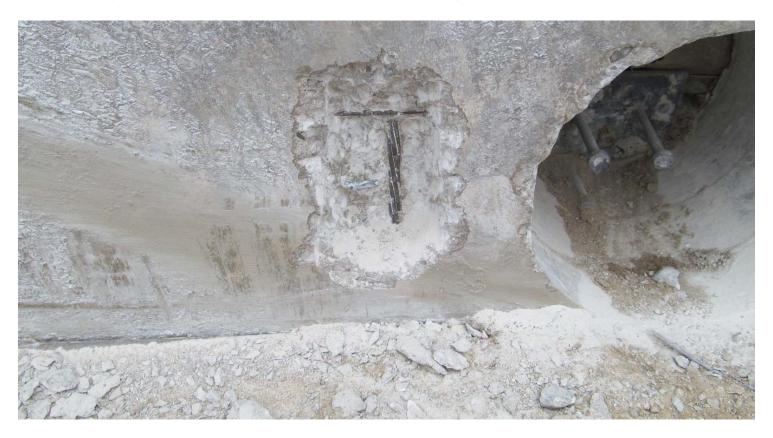
Photograph #13: The right-center prestressing strand was corrosion free. <sub>21</sub>
