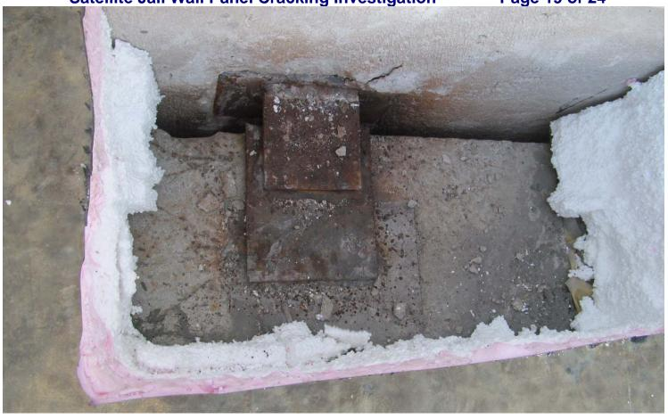
Photograph #28: Rust on roof plank / wall panel connection, East Wall
