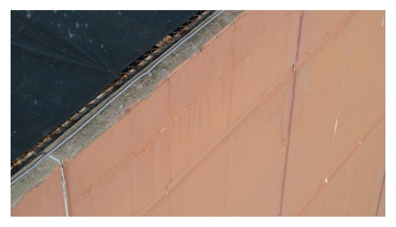
Photograph #24: East Exercise Yard Wall Cracking
