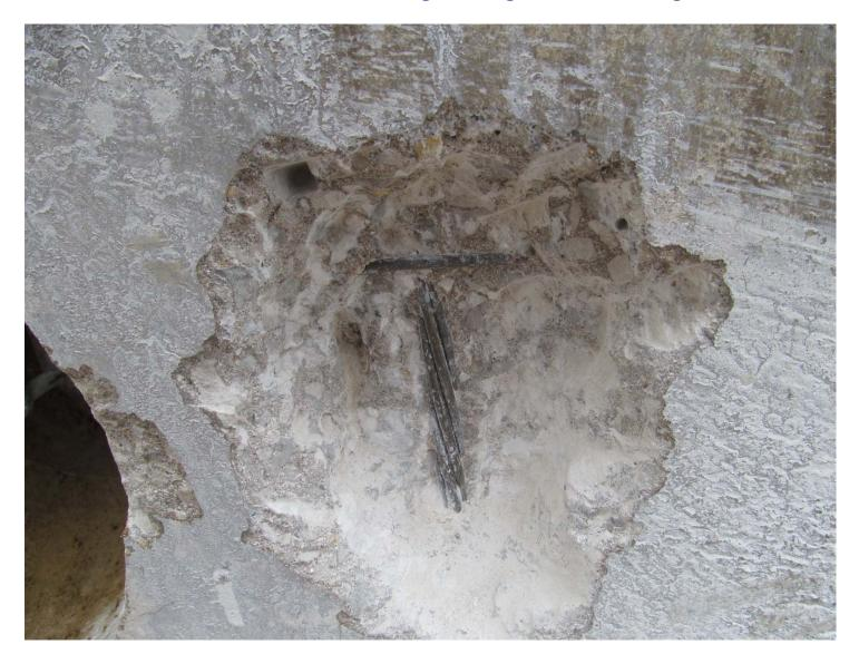
Photograph #18: The left-center prestressing strand was corrosion free.
