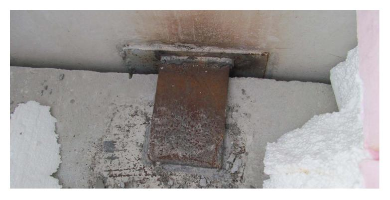
Photograph #29: Rust on roof plank / wall panel connection, SW Corner
