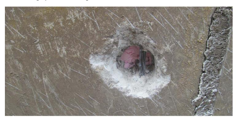
Photograph #20: The strand on the right side of the panel was corrosion free.
