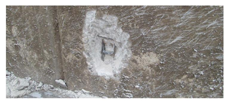
Photograph #11: The strand on the left side of the panel was corrosion free.<sup>20</sup>
