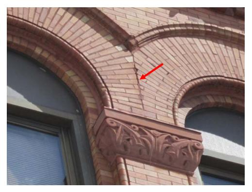
**Photo No. 3:** West façade third floor arched window head – open joints at brick masonry.
