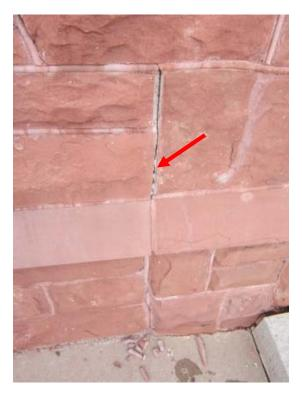
**Photo No. 4:** South façade sandstone building base – limited open joints at sandstone masonry.
