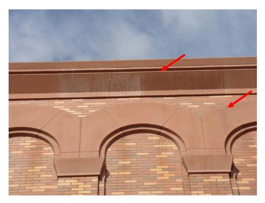
Photo No. 3: North façade cast stone cornice - staining.
