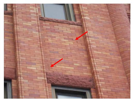
**Photo No. 1:** West façade spandrel area – typical area of step cracking with cracked brick and open mortar joints.
