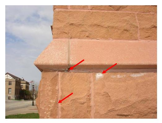
**Photo No. 1:** North façade cast stone base and horizontal band – minor cracked and open mortar joints and efflorescence. Note: Cast stone was used on the new addition to simulate cut natural stone.
