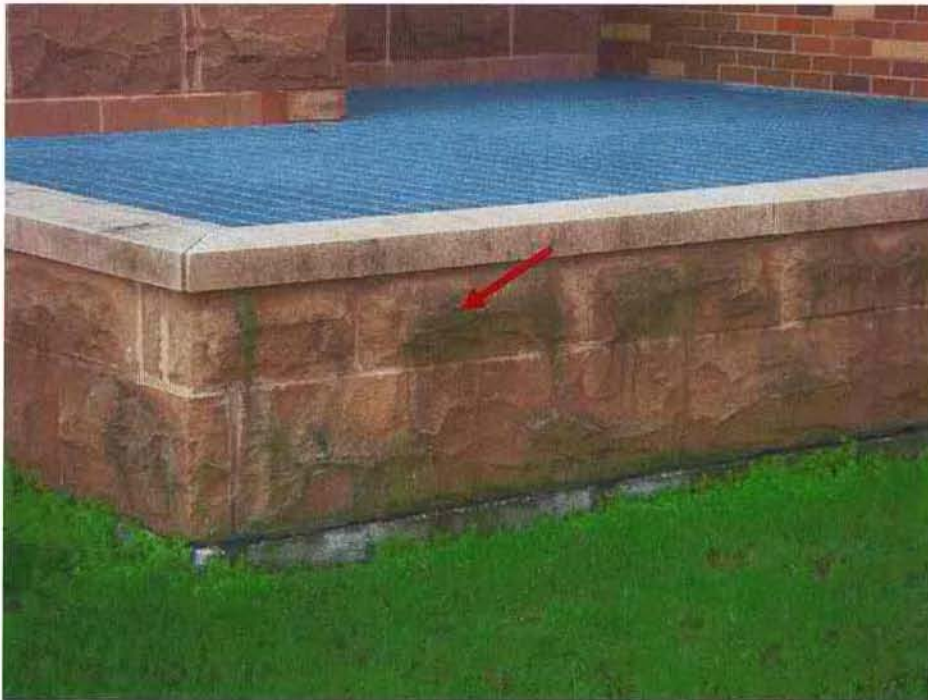
Photo No. 2: North façade cast stone wall with cap at equipment intake/exhaust – organic staining.
