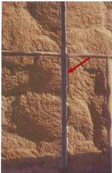
Photo No. 4: South façade cast stone building base – expansion joint sealant failure.
